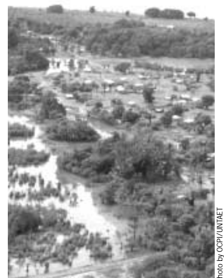
The aftermath of floods last year in Suai.
